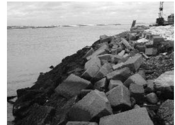
Riprap is commonly used to secure the shoreline where erosion is a problem.
